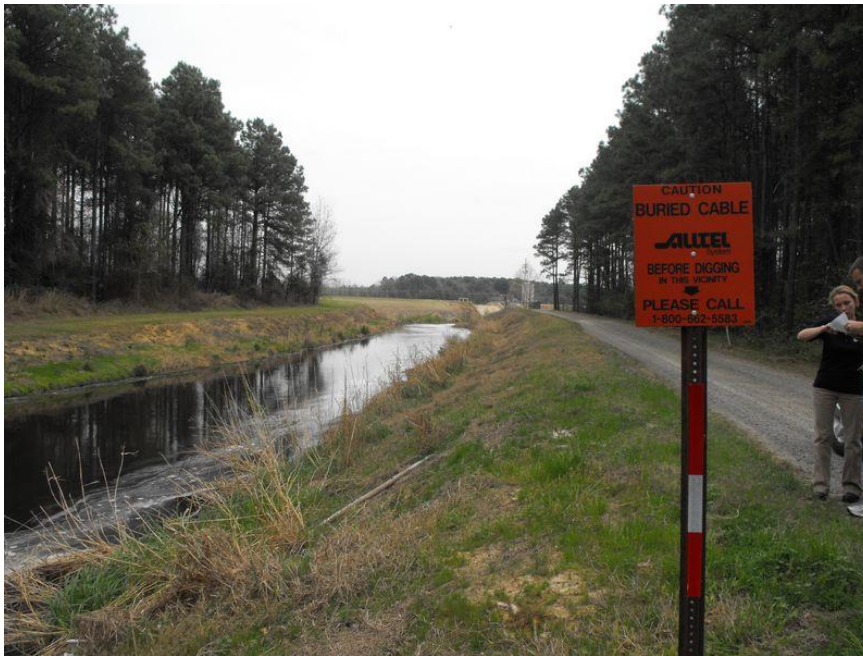
Near City of Crossett Discharge Pipe Looking Toward Surge Basin Discharge
