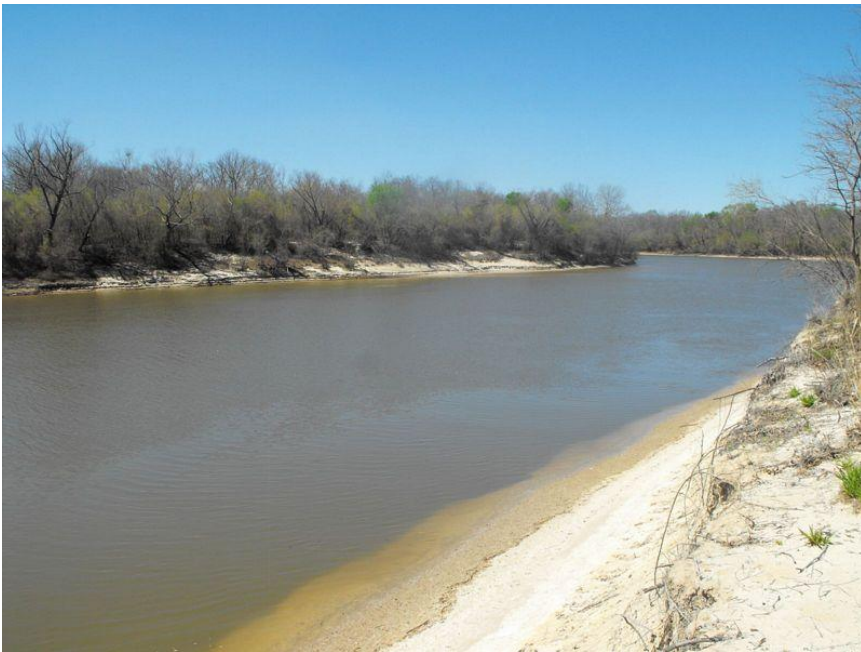
Looking Upstream on Ouachita River Near Confluence with Coffee Creek
