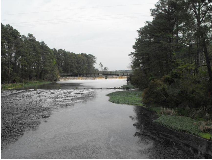
Looking at Discharge from Aeration Basin
