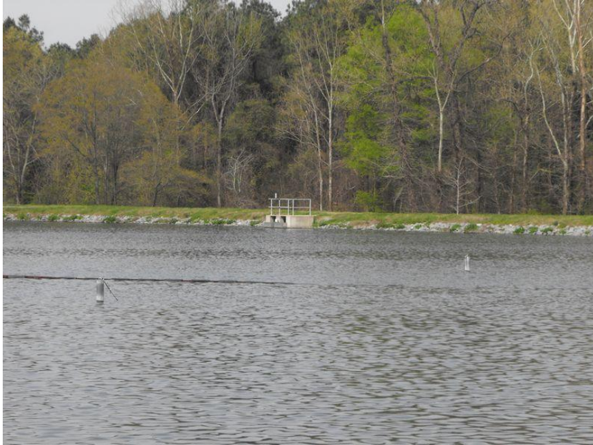
City of Crossett Wastewater Treatment Pond Outfall Structure from Across the Pond
