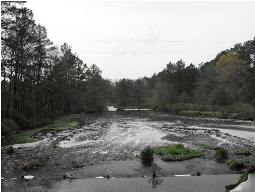
Looking Downstream on Aeration Basin Effluent Channel Toward Bridge
