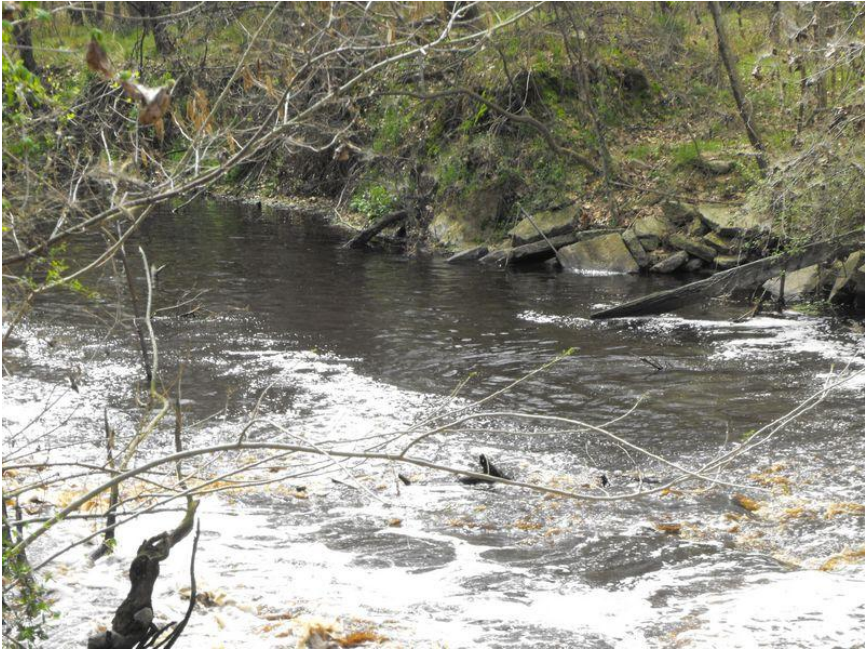
Foam Dissipation Immediately Downstream of Flume Turbulence
