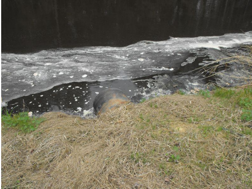
Discharge from City of Crossett's Pipe Entering Surge Basin Channel
